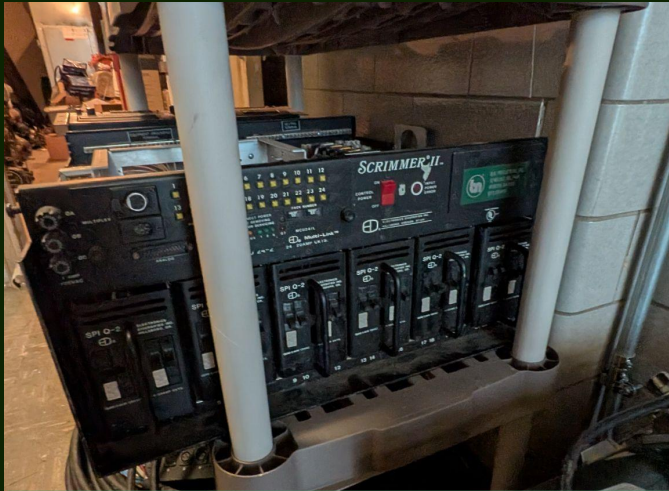
Removal of old dimmer rack
