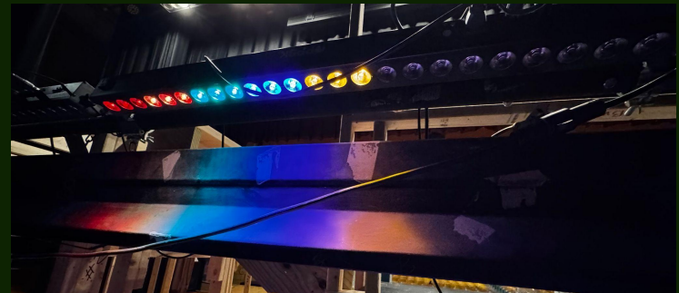
Installation of new cyc lights
